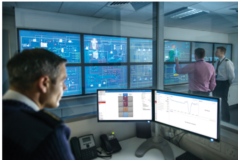
GearGard provides a history of the operating environment for NFPA 70B compliance.
